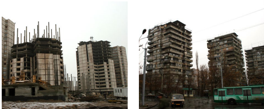
Construction, halted for decades; Housing near Yerevan
