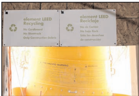
An example of the dumpster signage Tocci created to help subcontractors dispose of materials in compliance with LEED standards.
